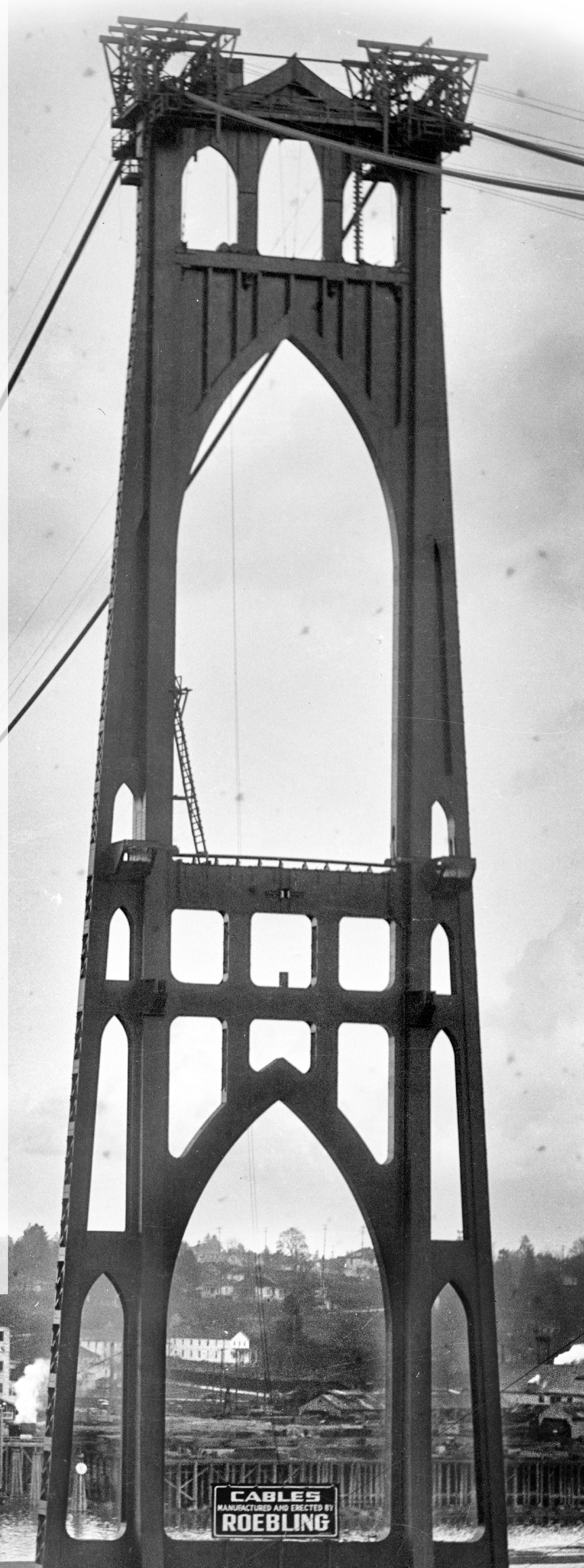
IBEW Local 48 apprentice electrician Eric Christenson Sr. started in the trade working on the St. Johns Bridge, shown in this 1930 photo awaiting suspender cables and the installation of its distinctive bridge deck and electric lamp posts. In 1945, Christenson would found his own firm, Christenson Electric. With its ubiquitous red trucks, NECA contractor Christenson Electric remains in operation today, in 2013, under its fifth owner.
