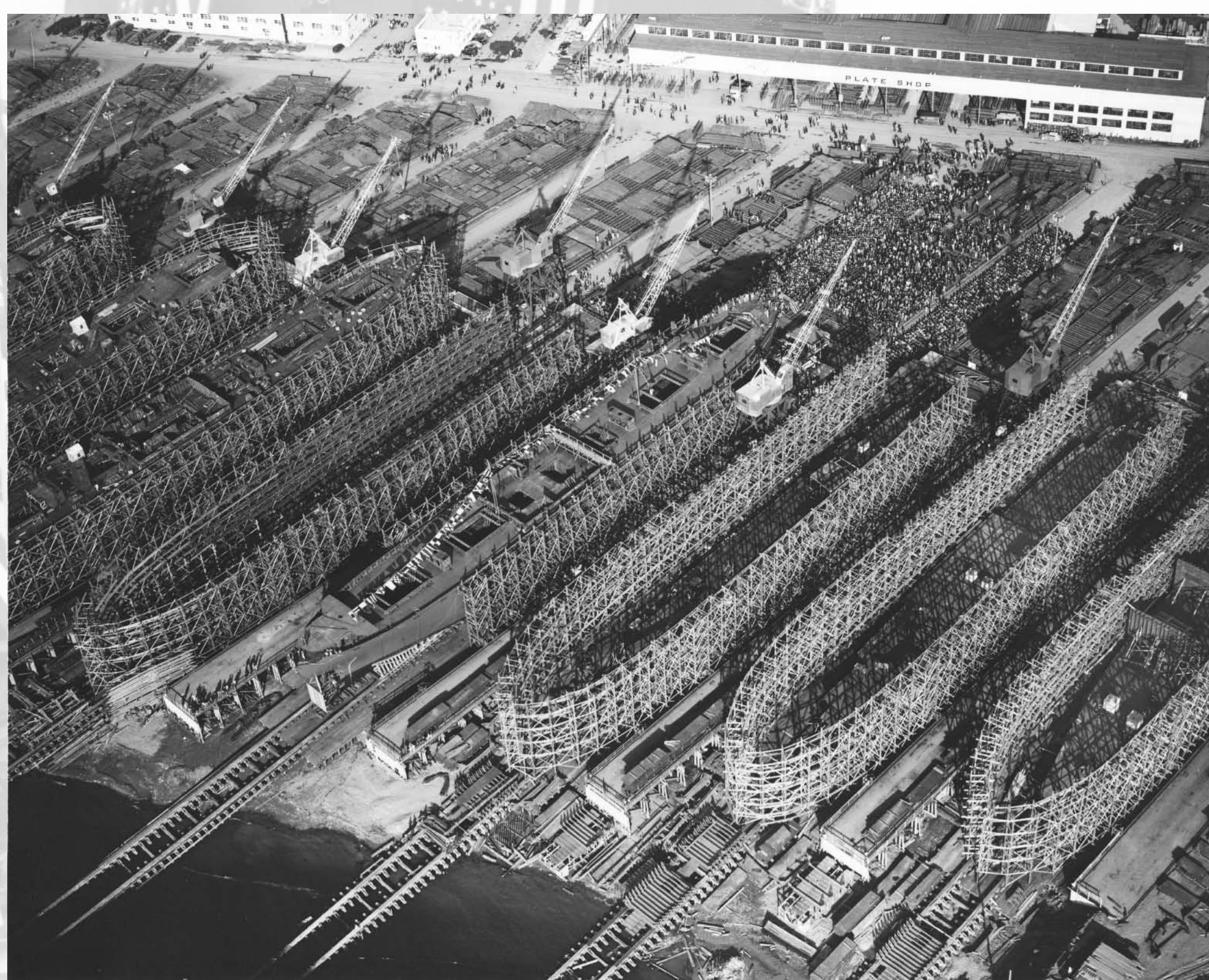
Henry J. Kaiser’s three Portland-area shipyards were “assembly line” operations comprising ships in varying stages of completion from keel block to finished hull at the moment of launching.
