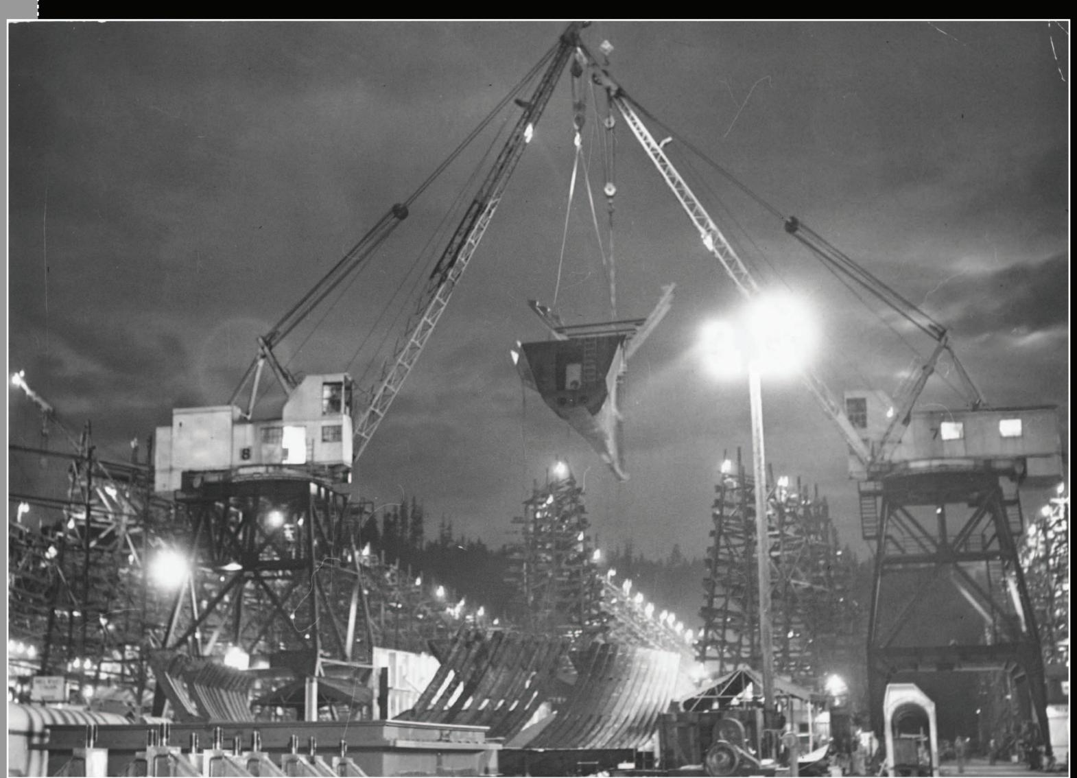
CRANES LIFTED AND SWUNG IN PLACE A PRE-ASSEMBLED 50-TON STERN UNIT IN A PORTLAND SHIPYARD, CUTTING TWO DAYS FROM LAUNCHING THE LIBERTY SHIP FOR WAR IN THE PACIFIC IN 1943:
